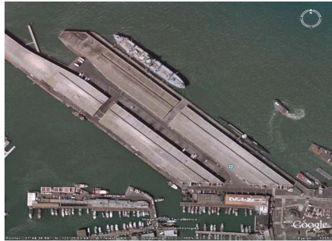
The Pier 45 Fish Processing Facility
